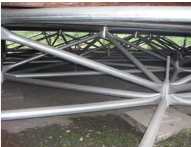
Public building on secure Tridetic foundation —Akiak
