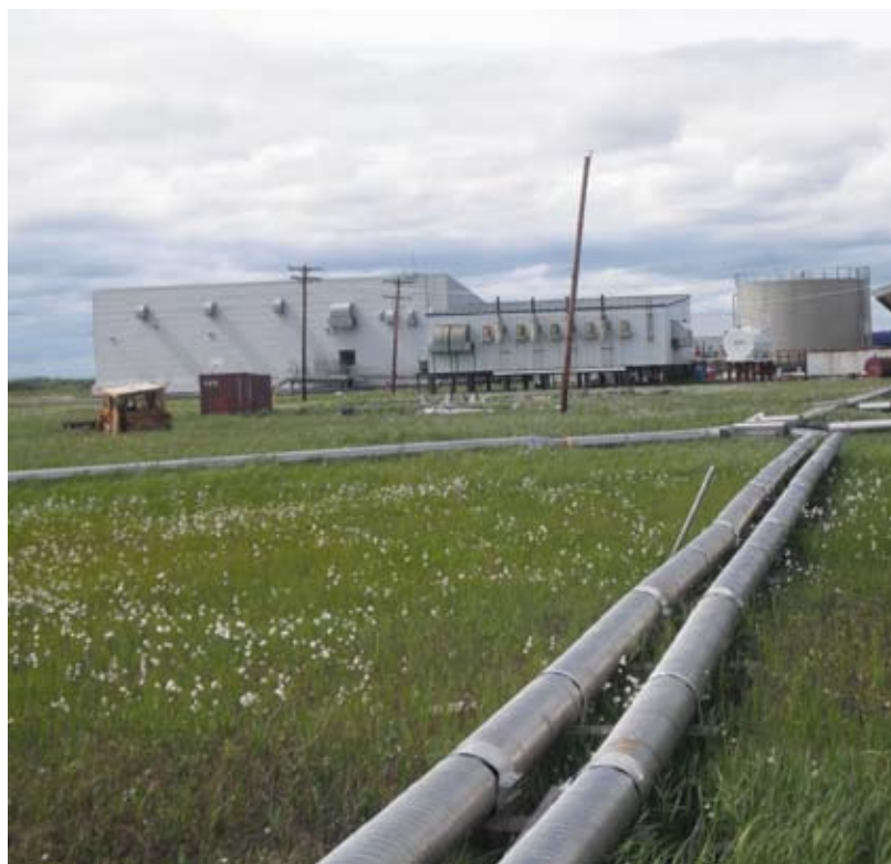
Water and Sewer arctic pipes secured on duckbill type ground anchors—Kotlik
