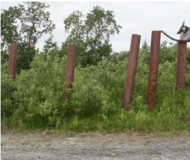
Steel pilings block river ice—Alakanuk
