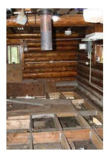
• Utilities – During repair or rebuilding, electrical wiring, junction boxes, switches, and outlets can be re-located to be above expected flood levels.
